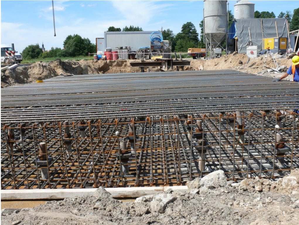
Fig. 8 Micropile foundation before being poured over by concrete
