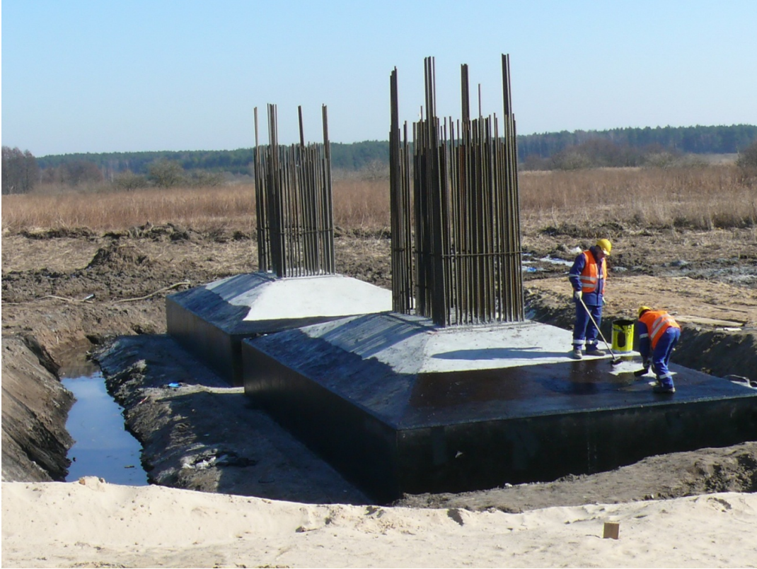
Fig. 9 Footing after pouring concrete
