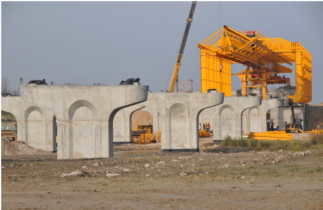
Fig. 10 Pillars ready for span concreting
