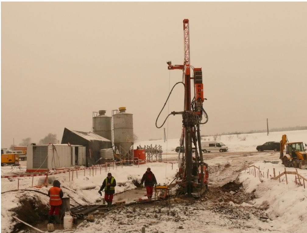
Fig. 7 Placement of micropiles, injection facilities in the background
